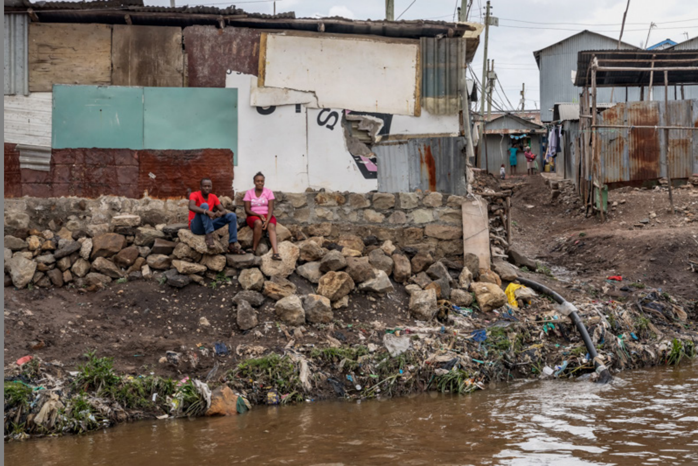
Lunga Lunga inhabitants on the banks of the heavily polluted Ngong River. The only bridge that allowed to cross it collapsed after a flood, causing further inconvenience to the inhabitants of the slum.
